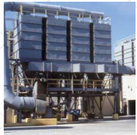
Baghouses and other advanced filtration systems prevent discharge of noxious, toxic or annoying fumes or odors.
